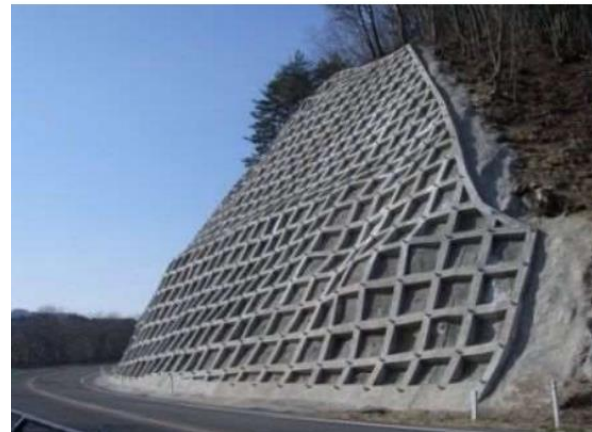
Fig. 1 Typical slope protection work
